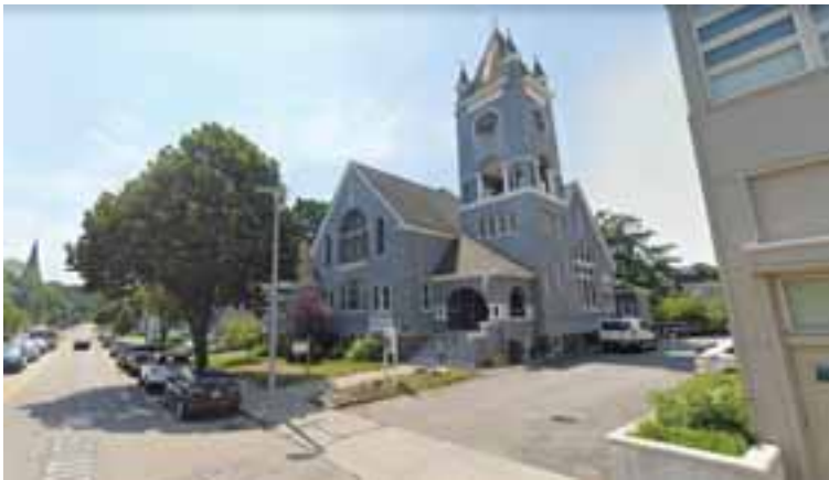
The Roslindale Congregational Church has decided not to open due to health and safety concerns.
