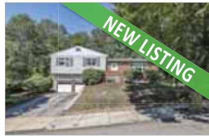
69 HACKENSACK ROAD WEST ROXBURY $789,000 Listed by David Greenwood
