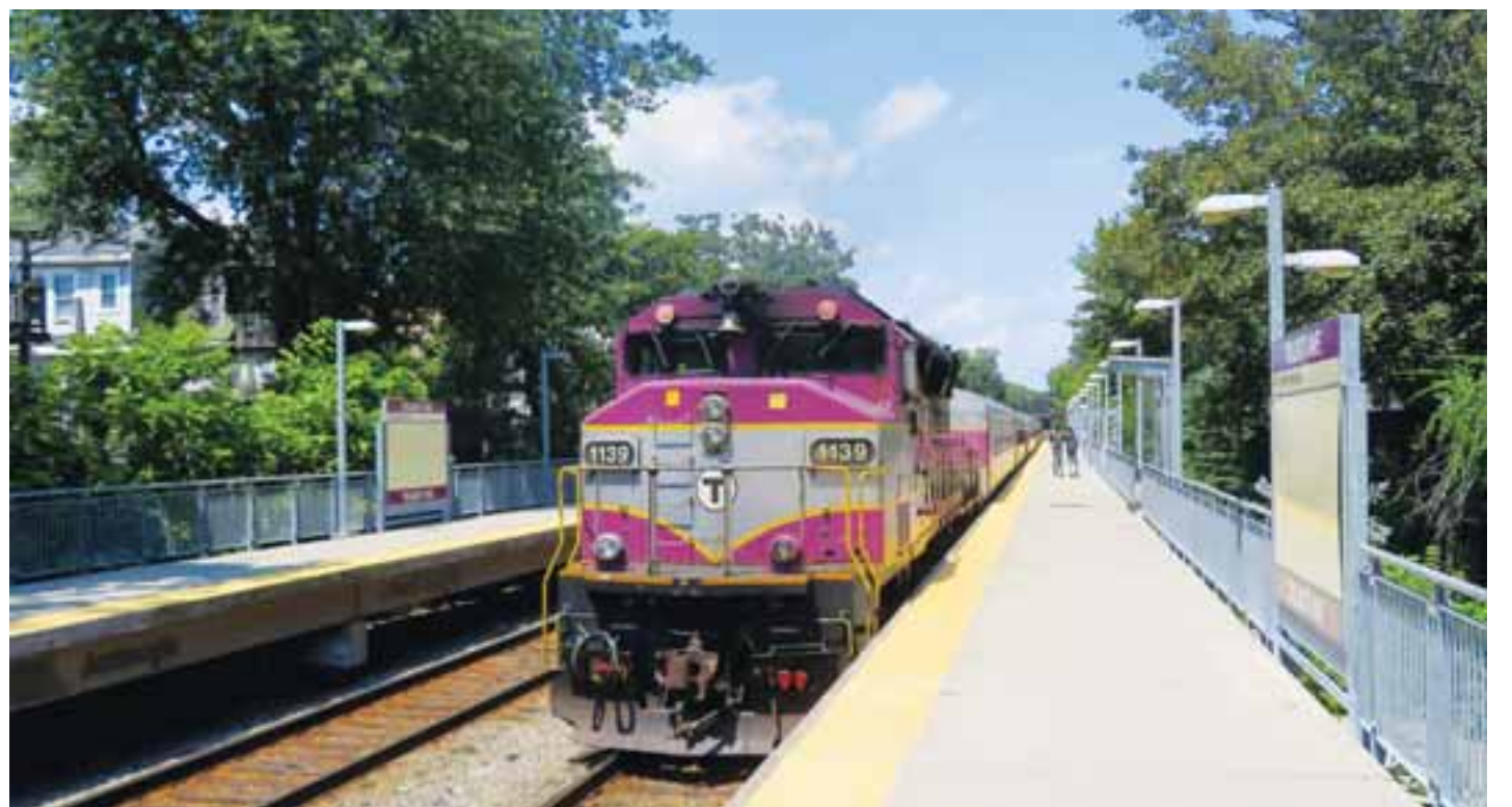
Residents and organizers are pushing for legislation to electrify and increase the frequency of trains on the Fairmount Line.
