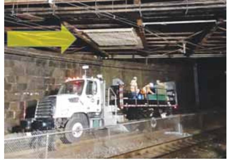
Work is progressing on the bridge project, if a bit slower than residents would probably like.
