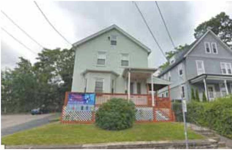
The ZBA denied an application to add three units to this building because of unit size problems.
