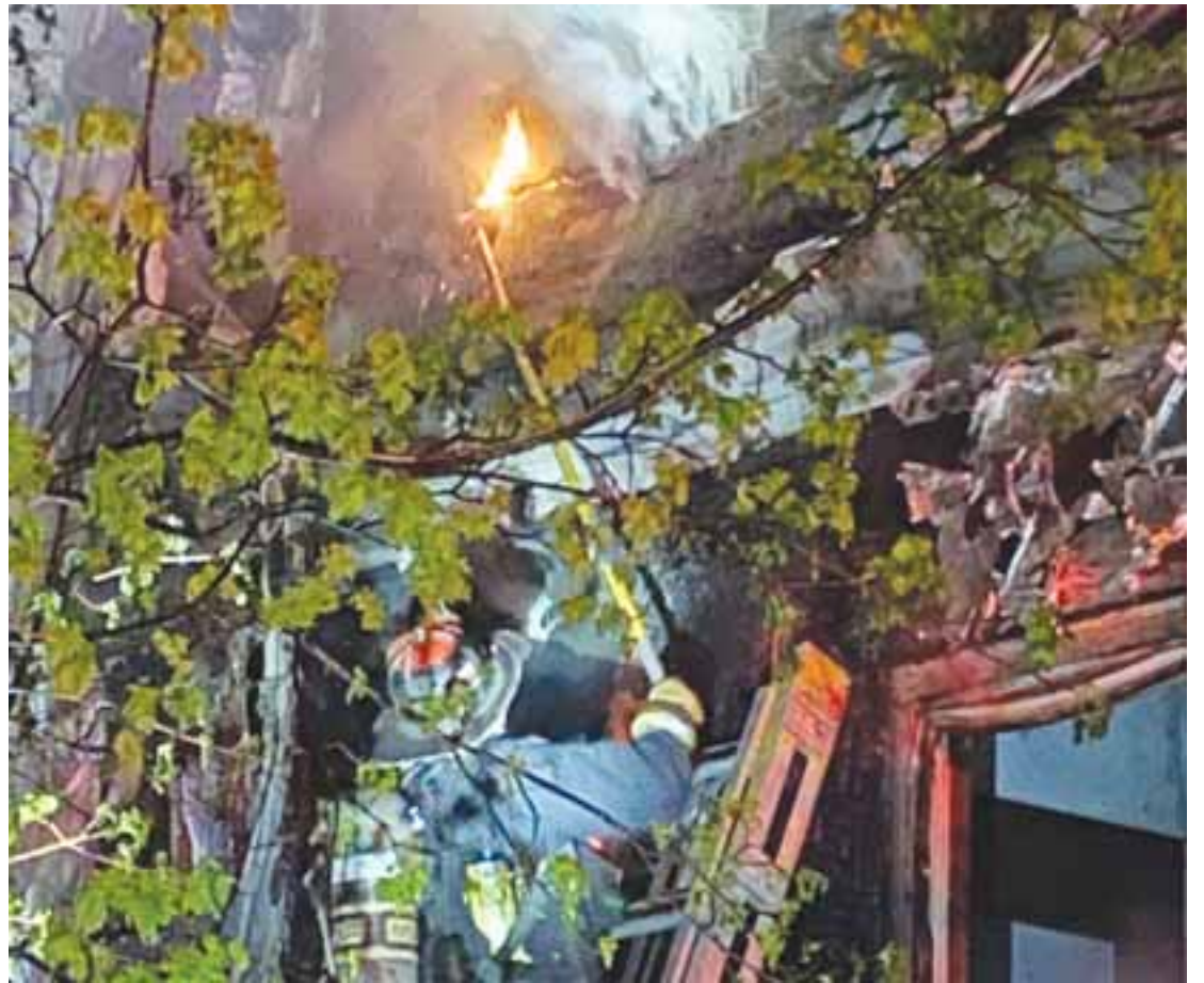
The Boston Fire Department reported they responded to a fire at 3:10 a.m. at 260 Cummins Hwy. in Roslindale. The two-and-a-half story building took about two hours to fully knock down, and the damage was estimated at $150,000. The Fire Investigation Unit stayed on scene to try to determine the cause of the fire.
