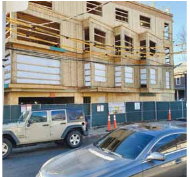
The dispute regarding 11 Dana Ave. enters what might be its final chapter after the ZBA ruled last week that the project is as-of-right.
