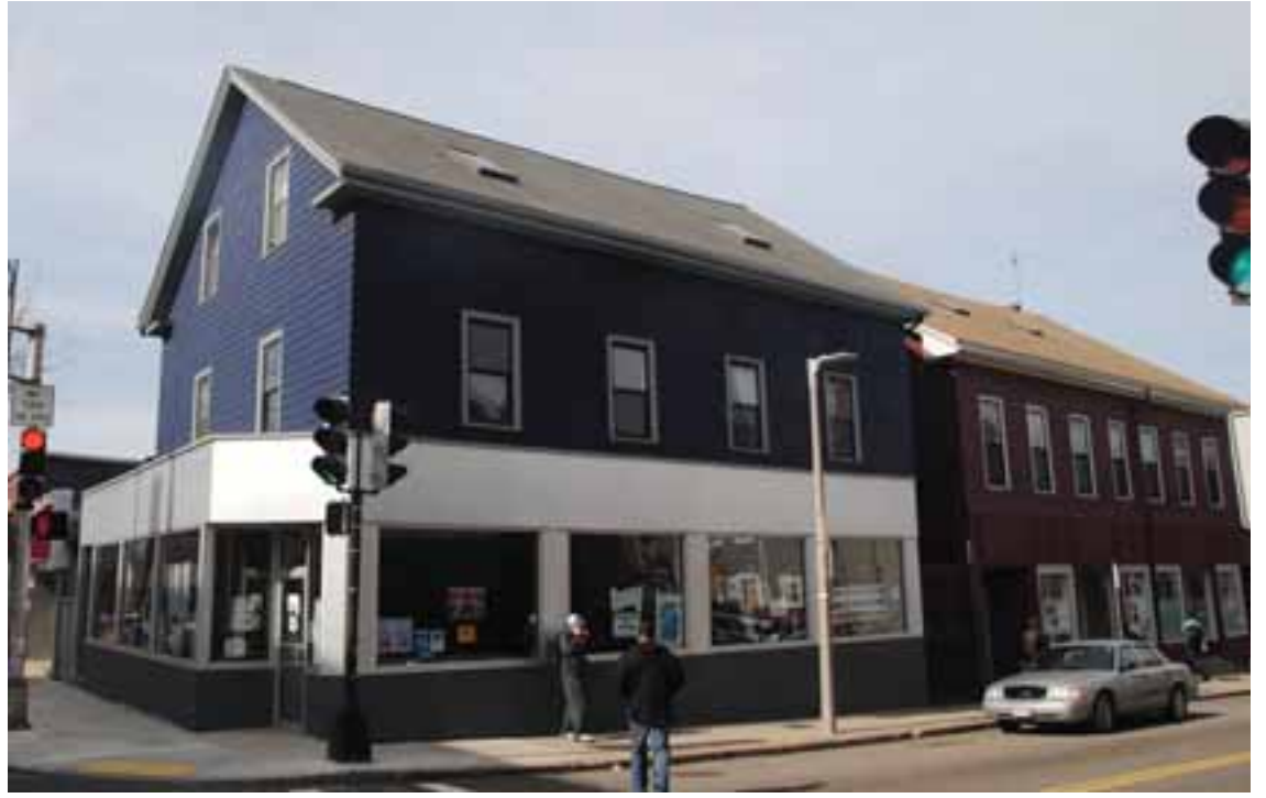
3353 Washington St./211 Green Street will remain standing for two more years as BCV received an extension on its development of the property.
