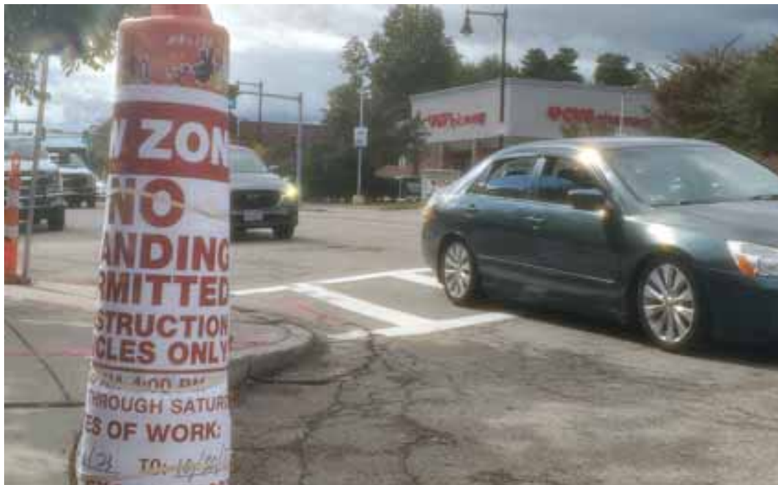
Road work has started on Centre Street in West Roxbury for the safety redesign and lane reduction of the street.
