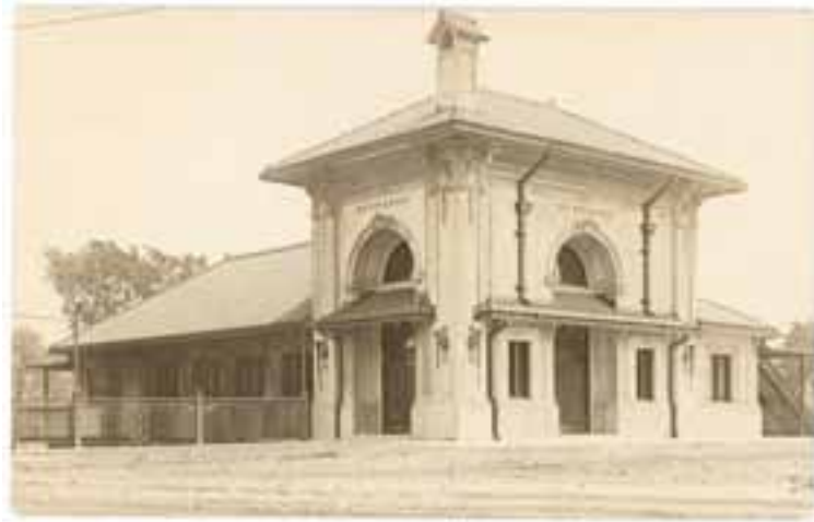
Several carvings believed to be from this Hyde Park rail station are set to be placed and restored at the HP Library with CPA funds.
