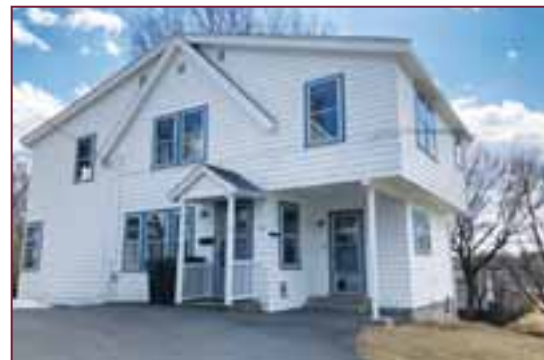
28 ROBINWOOD ROAD, DEDHAM
