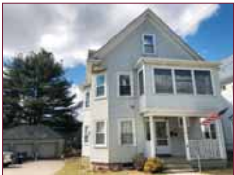
17 CENTRE TERRACE, WEST ROXBURY
