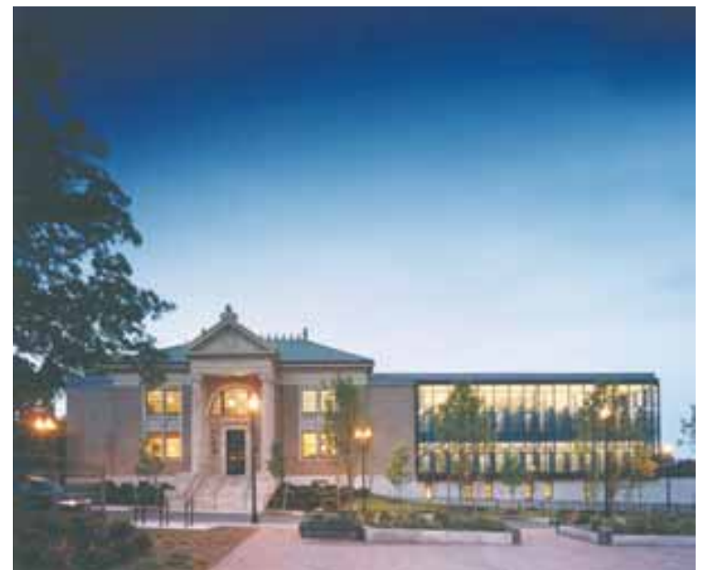
The original, left, and the 20-year old addition, right.
