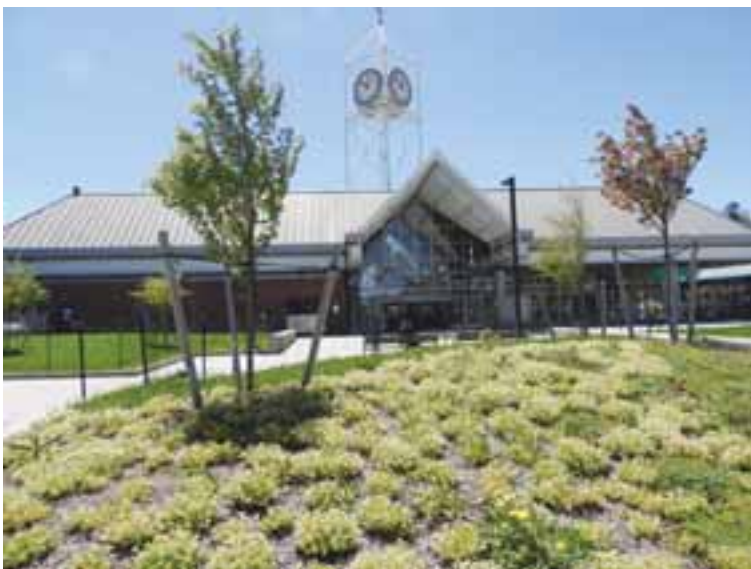
Groundcover beds and new trees were planted at the Forest Hills Station Plaza.
