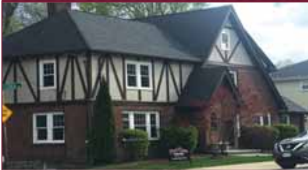
1658 CENTRE STREET, WEST ROXBURY
