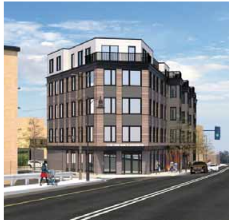
The current doctor’s office is planned for apartments above, and developers now propose to take over the adjacent mechanic shop.
