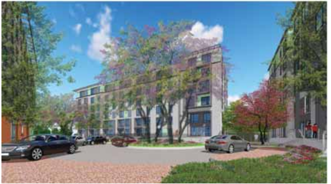
The interior court of the Residences at Forest Hills will be built over the Stony Brook culvert.
