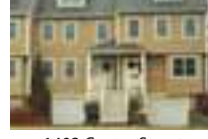
1403 Centre Street West Roxbury
