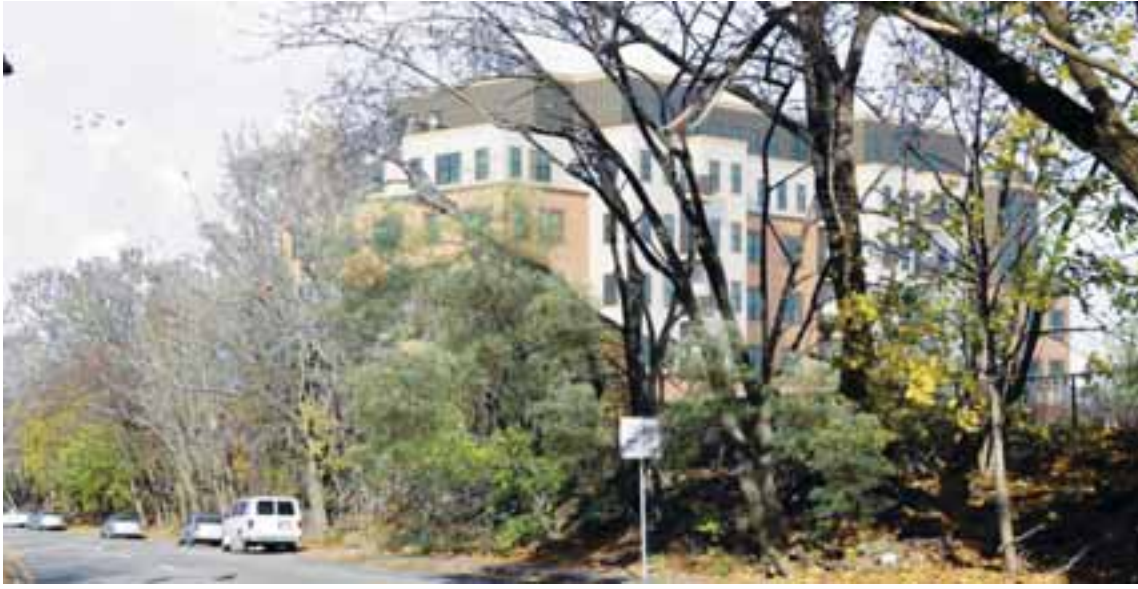
Residents were concerned about drainage and parking for the project.
