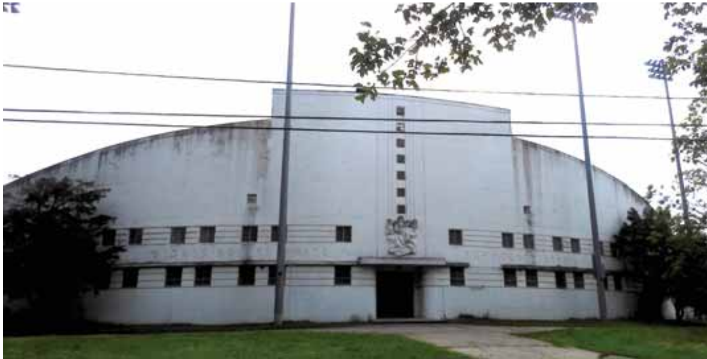
A view of the west grandstand that is proposed to be leased to Boston Unity Soccer.
