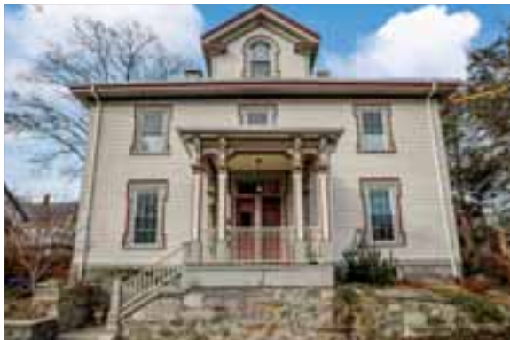
10-12 HILBURN PLACE, ROSLINDALE
