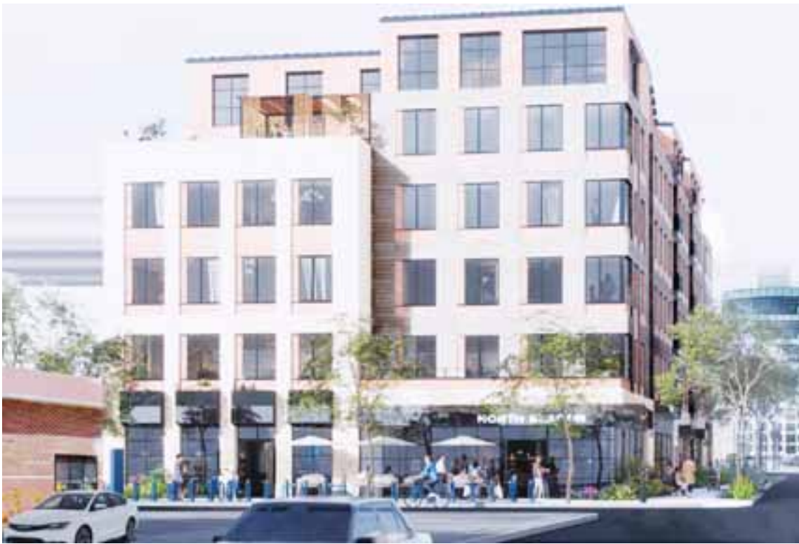
Residents had concerns regarding the proposed project at 131 North Beacon St., but most of the discussion was positive.
