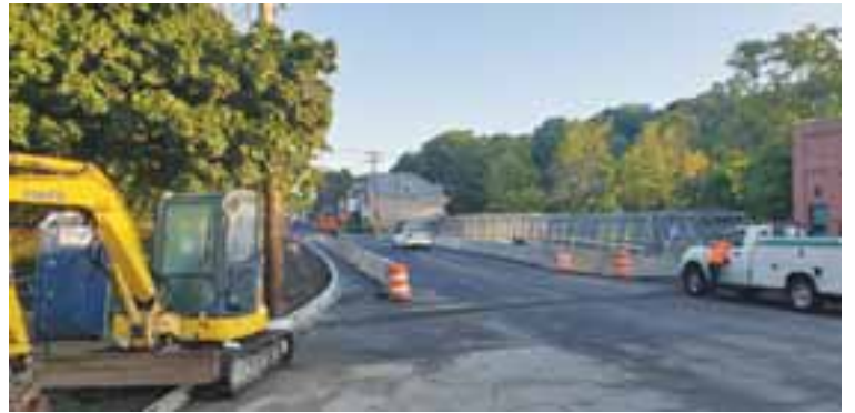
Work is still ongoing, but the bridge itself is ready to handle whatever traffic you can throw at it.
