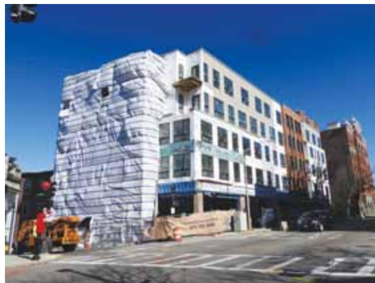
Tempo at 3193 Washington Street at Montebello Rd. City Realty has stopped construction.
