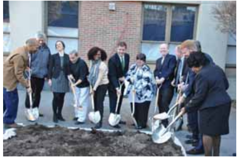
Ground breaking ceremony in the outside courtyard. Center: Mayor Walsh, flanked by Gina Rector (R) and Natacha Dunker (L), board chair of Urban Edge. BHA Director McGonagle is behind Rector.
