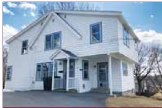
28 ROBINWOOD ROAD, DEDHAM
