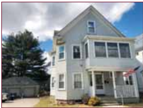
17 CENTRE TERRACE, WEST ROXBURY
