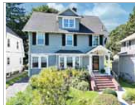
287 STRATFORD STREET WEST ROXBURY
