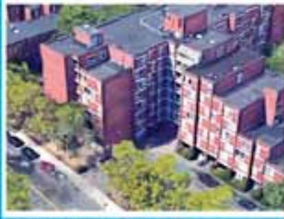
Existing Building & Site
