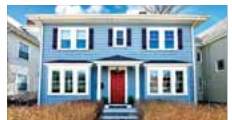
1694 CENTRE STREET, WEST ROXBURY
