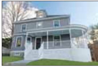
12 WESTMOUNT AVENUE WEST ROXBURY
