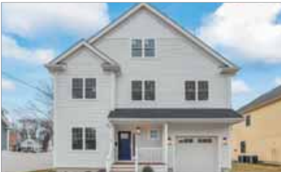
24 BELLE AVENUE WEST ROXBURY
