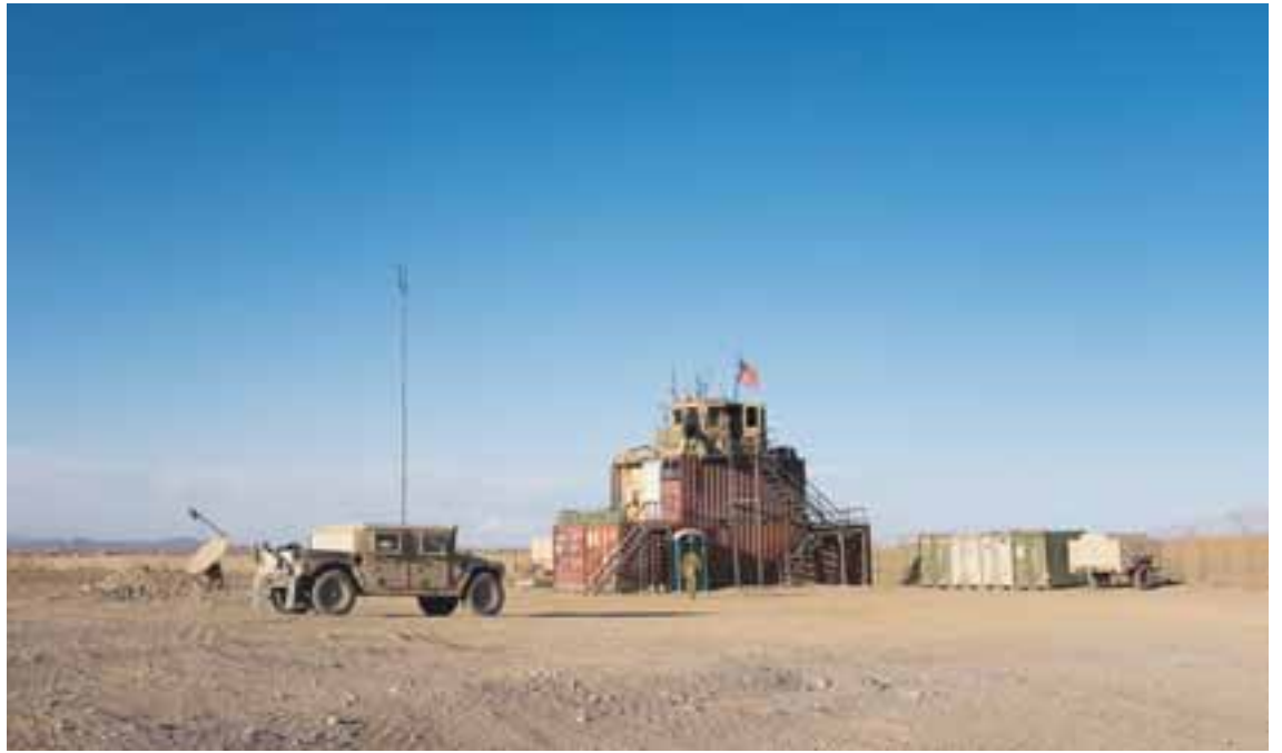
One of Dinner's displayed pieces was of the Air Traffic Control Tower in Dahlke, which was built from spare shipping containers by the 101st.
