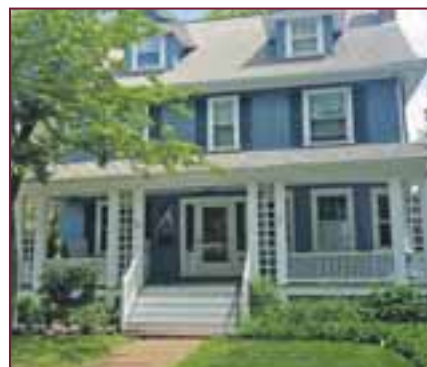
71 HASTINGS STREET, WEST ROXBURY
