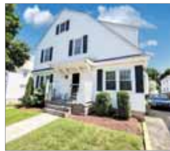
39 AVALON ROAD WEST ROXBURY
