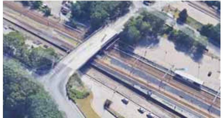
This spring will see the return to work on the bridge and the signalization of its two intersections.
