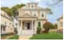
44 Lorraine Street Roslindale
