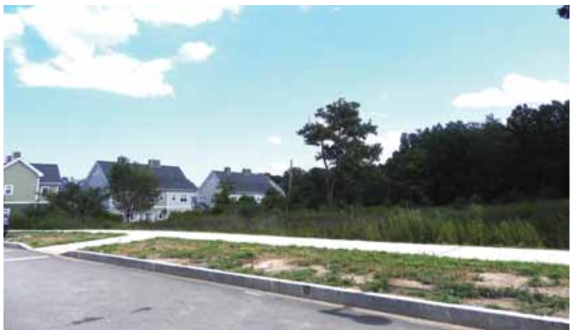
The site of the planned Russell House, which will have four stories and 48 mixed-income homeownership units.
