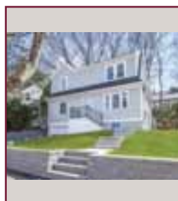
110 Dwinell Street West Roxbury
