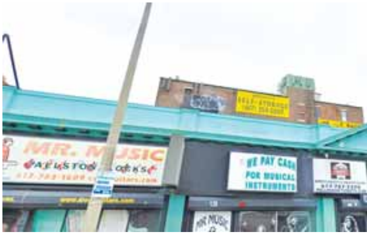
Located just behind Allston's iconic Mr. Music shop on Harvard Avenue, the old Yellow Brick Self Storage Building is slated to become the new home for recording studio and practice space provider Studio 52
