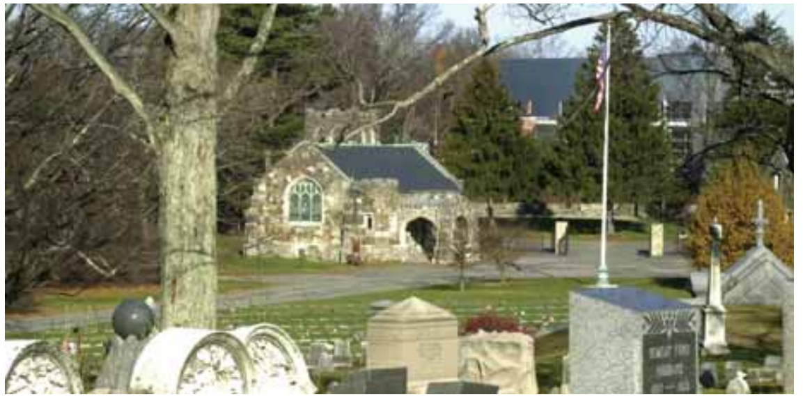
The Mount Hope Cemetery will be getting a face lift, along with its administration building.
