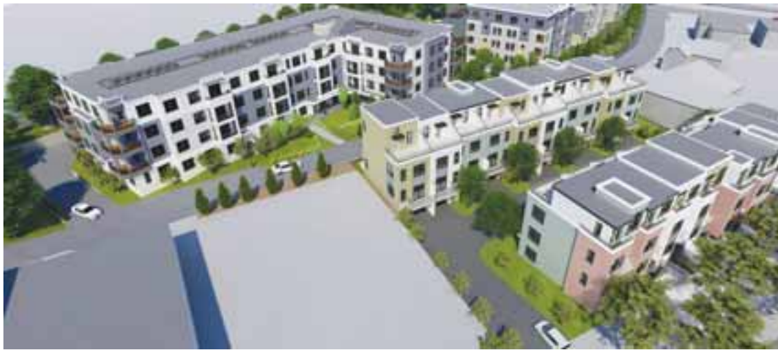
The development will combine four parcels off of the VFW Parkway to compliment the Oak Row development on 1235 VFW already approved by the BPDA.
