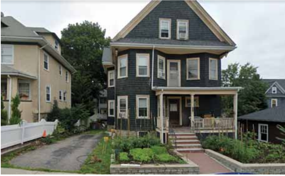
This house at Colberg Avenue in Roslindale will now be officially labeled as a three-family.
