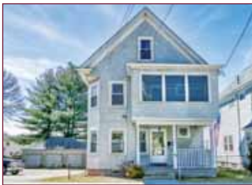
17 CENTRE TERRACE, WEST ROXBURY
