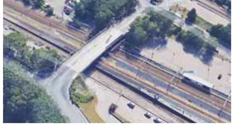
This spring will see the return to work on the bridge and the signalization of its two intersections.
