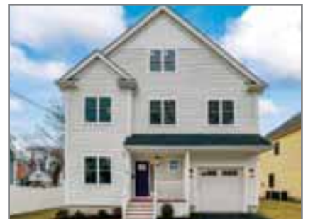
24 BELLE AVENUE, WEST ROXBURY
