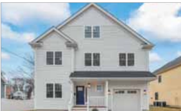
24 BELLE AVENUE WEST ROXBURY
