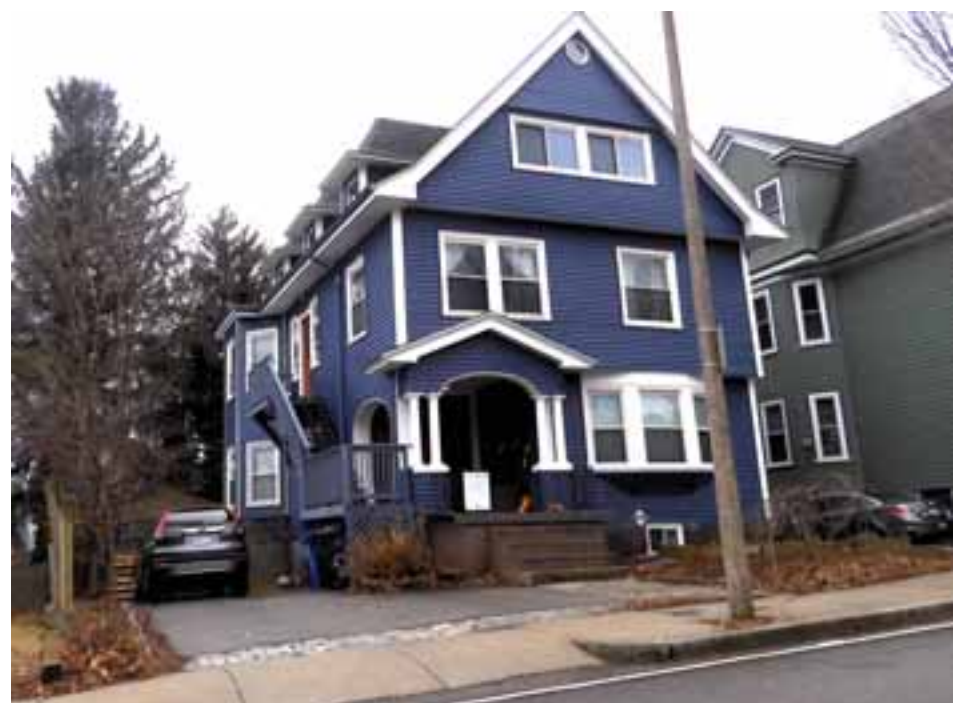
The owner of this house is looking to create a new unit out of the garage behind the main structure at 294 South St. in Jamaica Plain.
