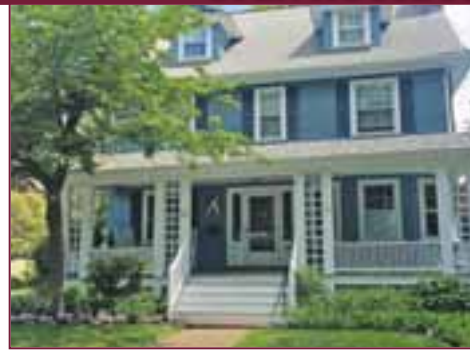
71 HASTINGS STREET, WEST ROXBURY
