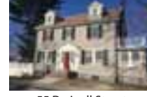
55 Dwinell Street West Roxbury
