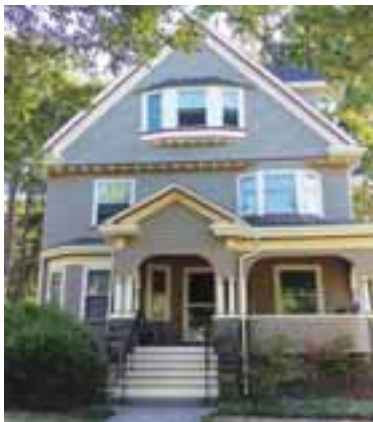
33 Stratford Street, West Roxbury, MA 02132
